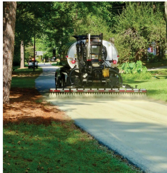
Picture 1: Photocatalytic pavement treatment in Raleigh, NC
