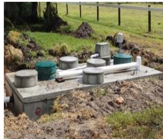
ATU with built-in Trash Trap
